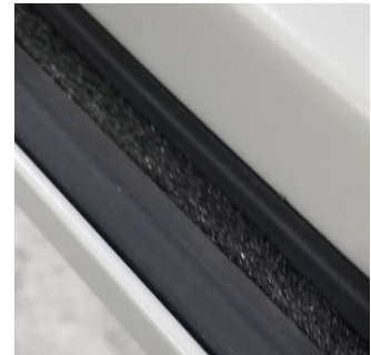
Double Magnetic Seals at Head and Jambs
