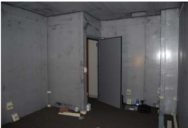
EM-S chamber under construction.
