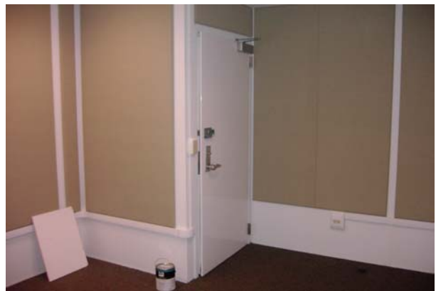
EM-S chamber at commissioning.
