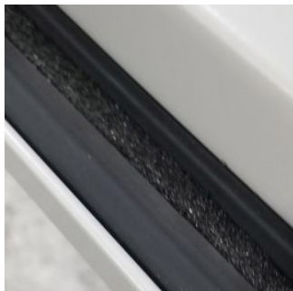
Double Magnetic Seals at Head and Jamb
