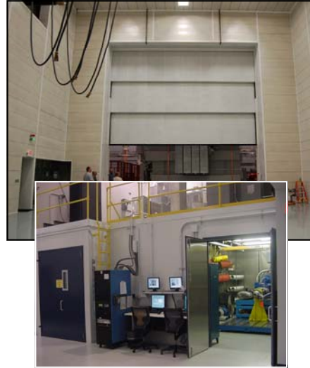
QuietMod™ Acoustical Test Facilities
