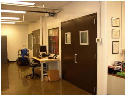
6' x 7' STC 52 Double-Leaf Door with 12" x 12" double glazed windows. New York, NY
