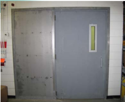
4' x 8' STC 50 Single-Leaf Door with 4" x 25" ADA window and 3' x 8' filler panel. Fond du Lac, WI
