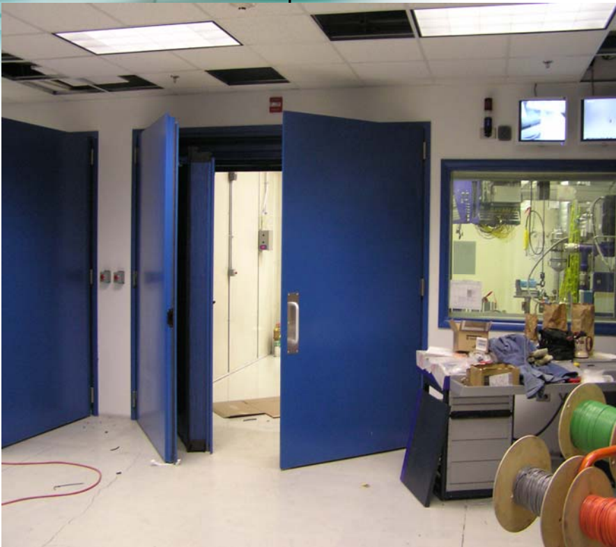
8' x 8' STC 48 Double-Leaf Door piggy-backed onto larger STC 60, fire rated, projectile rated, blast rated door—paired with an STC 62, projectile and blast resistant 4' x 8' window system. Wixom, MI
